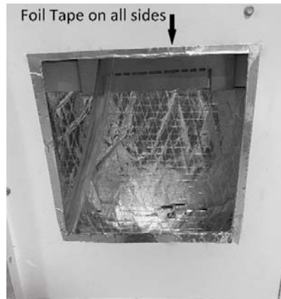
FIGURE 7: PLENUM OPENING WITH TAPED EDGES
